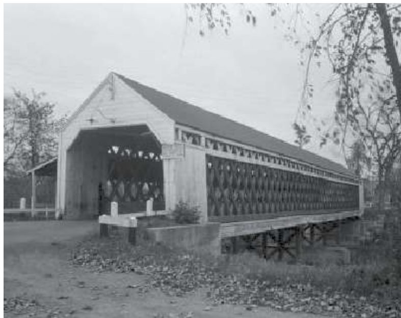
Nehemiah Jewett Bridge, photographed by Frank O. Branzetti for the Historic American Buildings Survey, Oct. 17, 1940
